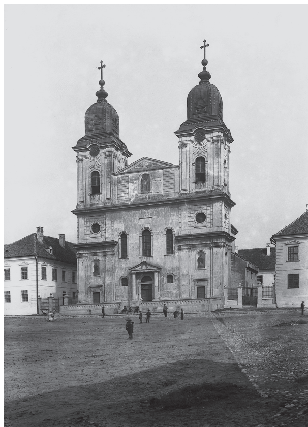
Fig. 7. Main façade of the Cathedral of Blaj in the early twentieth century (Budapest, Forster Gyula National Centre for Cultural Heritage Management, Photo-archive 33540N)
